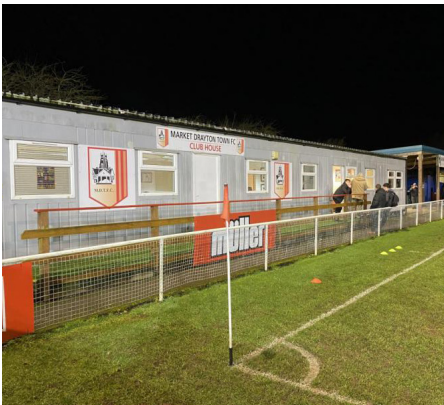
Electrical works completed in club house.
