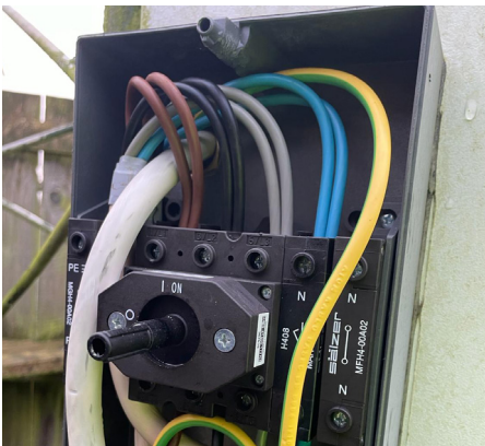
Outdoor electrical remedial work.
